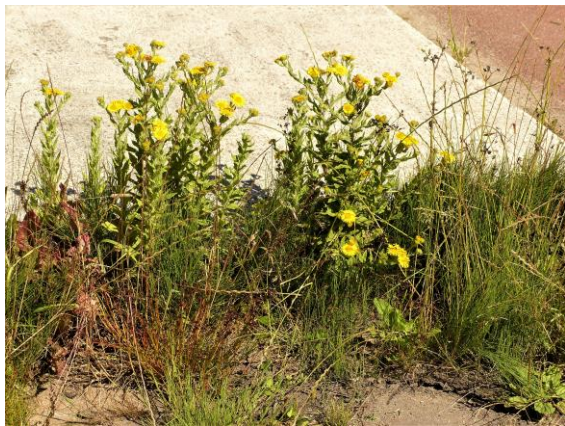
Heelblaadjes in beton (Fred)
